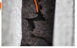
Classic UV damaged tar paper. Once the roof decking is exposed below, leaks begin.
