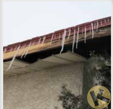
SOFFIT DAMAGE
