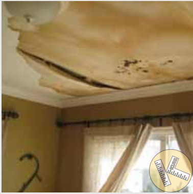
WATER DAMAGE
