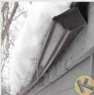
GUTTER DAMAGE
