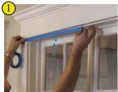
Determine where the water is leaking through the frame. Dry the area as much as possible; quickly apply some masking tape as shown.
