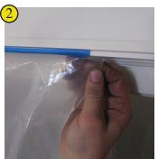
Apply the top half of the tape to the door/window frame so that the bottom half (along its length) is left exposed. This is what you will stick your plastic/aluminum foil to.
