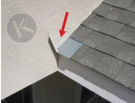
Samples of kickout flashings. Top, a kickout flashing installed in a cedar shingle sidewall. Below, a kickout installed in a stucco wall. Notice that one drains into a gutter and the other doesn't. Both are common in Minneapolis homes.
