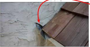
Here is a sample of a kickout flashing installed into an existing stucco wall, under a new cedar shake roof in Minnetonka, Minnesota. It is possible to use a ultrasonic saw to carefully kerf into an existing stucco wall in a way that allows one to insert a kickout flashing under certain circumstances. Other times we need to remove stucco and patch the area after the kickout is installed.
