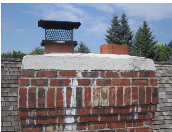
Chimney cap repaired via the application of magic goop. This 'ten year fix' lasted two years. We replaced the chimney crown entirely.
