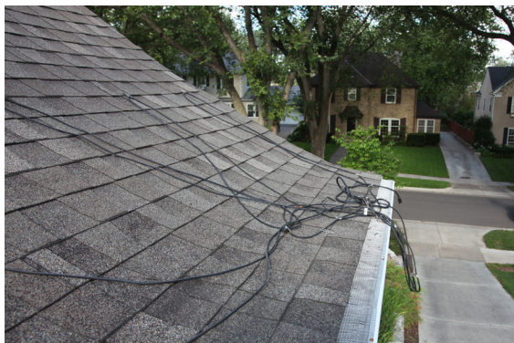
Heat cable job on Edina Country Club home. Cheap cable bought from Home Depot. Spaghetti install method used.
