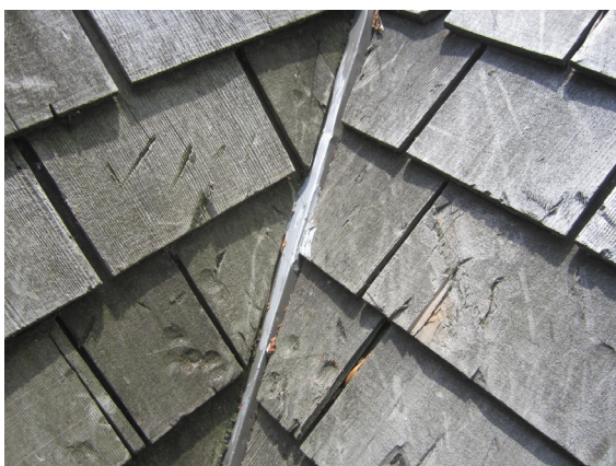
Roof damage caused by ice dam removal with a hammer and pick in Edina. The valley metal was punctured in many locations. Ouch.
