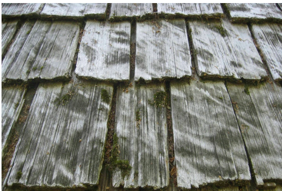
Cedar roof washing attempted on roof that should never have been washed. We ended up replacing this roof.
