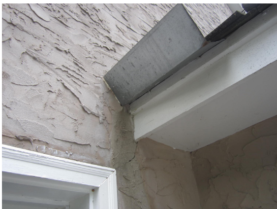
Kickout flashing installed on cedar roof in Minnetonka. It was not installed into the stucco and was therefore useless.
