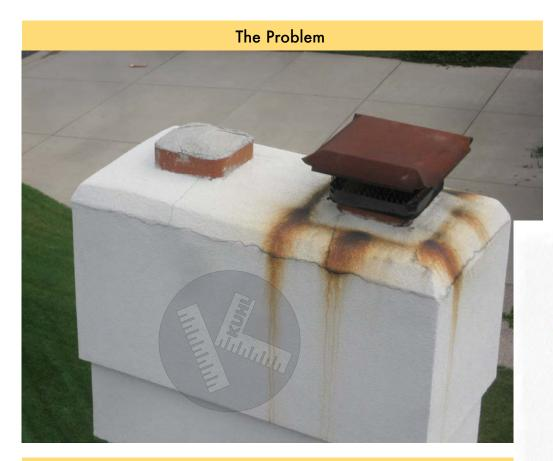
The cap of the original chimney had a sloped mortar core with a top coat of stucco (portland cement). Bad idea. We don't like stucco to be used on horizontal surfaces unless particular steps are taken. Water was leaking down into the chimney column and causing trouble below. Instead of rebuilding the upper portion of the chimney (big bucks) we advised our client to cover the existing cap with a custom copper chimney cap.
