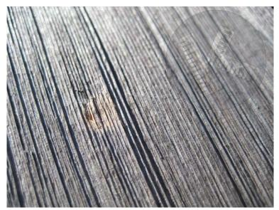
This is an impact mark from a .75" hail stone on a 3 year old medium hand-split cedar shake roof in Edina, Minnesota. Such hail frequently causes severe damage to cedar shake and shingle roofs. In this case the wood was resilient enough to escape with only a minor ding. Neighbors all around this home had their roofs replaced from the same hail storm. This roof sustained only cosmetic damage.
