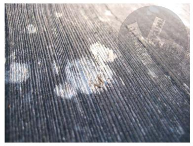
Here we see a 13 year old hand-split heavy cedar shake roof with heavy black mold and oxcidation. The direction of the hail storm resulted in glancing blows rather than perpendicular strikes. The discoloration on the surface of the cedar shake has been removed by the impact of the hail stone but no functional damaged was done that will affect the integrity of the shake.
