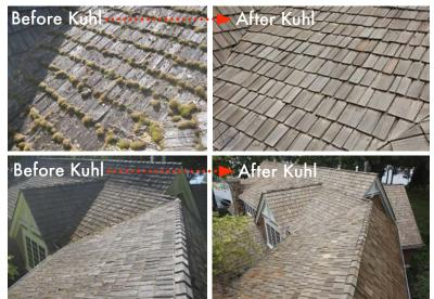
Before and after cedar roof cleaning, repairing and preservation. This roof was 17 years old.
