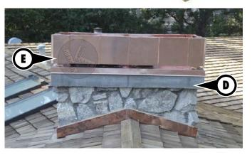
After forming and pouring the new chimney caps (D) we designed and installed the copper chimney shrouds (E). Each chimney shroud accommodates the exact dimensions of the cap beneath as well as the different flue penetrations. We wrapped the copper up and into each clay flue to keep water out of the system completely (F). The resulting chimney treatments look phenomenal from the curb and will keep the home free of leaks for years to come.
