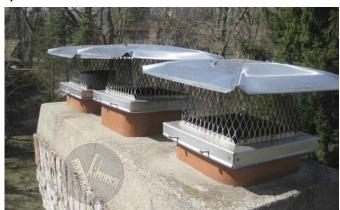
Installing the typical steel chimney cap, such as the ones shown here, ranges from \$125-350 per location depending on flue size and height off the ground.
