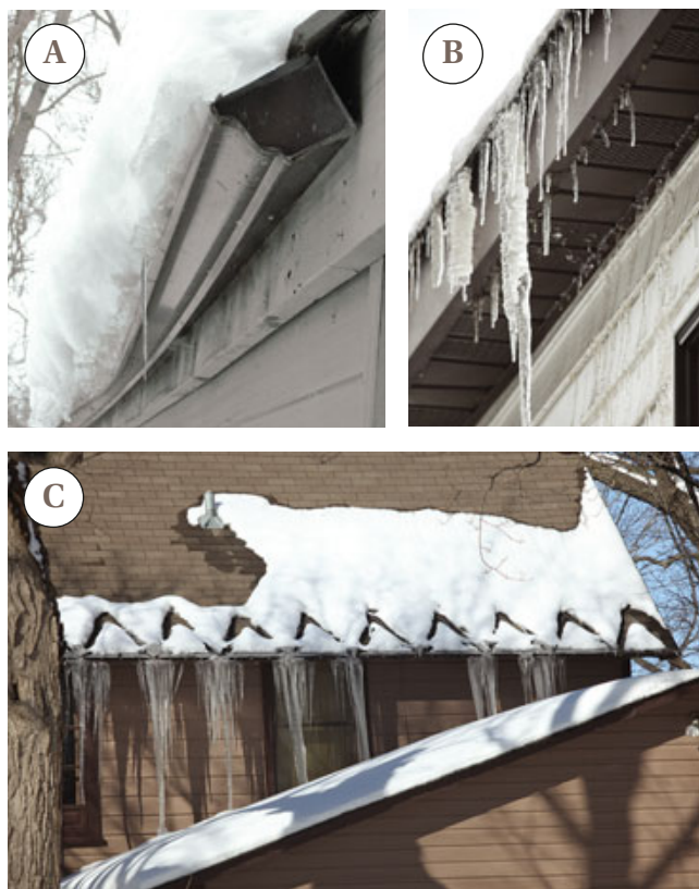
Figure 3. While gutters are often damaged by ice (A), they are not the cause of ice dams (B), as is commonly thought. Another misconception is that electric heat cables can prevent ice problems (C). Besides being largely ineffective, heat cables consume a lot of electricity and can burn out quickly.
