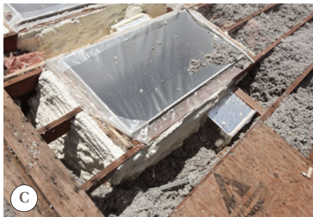
Figure 5. Inadequate insulation (manifested here as lines of snowmelt along the rafters), a narrow, poorly ventilated soffit, and heat loss around the skylight all contributed to ice dams on this house (A). Low-slope roofs, like the one on this shed dormer (B), are commonly plagued with ice dams. In this retrofit job, the author has used two-part spray foam to thoroughly seal and insulate a pair of skylight wells (C).
